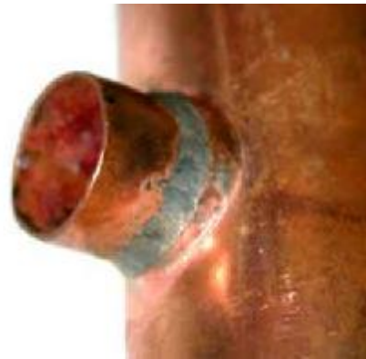
Close up of brazed header joint (CuP6 brazing rod)
